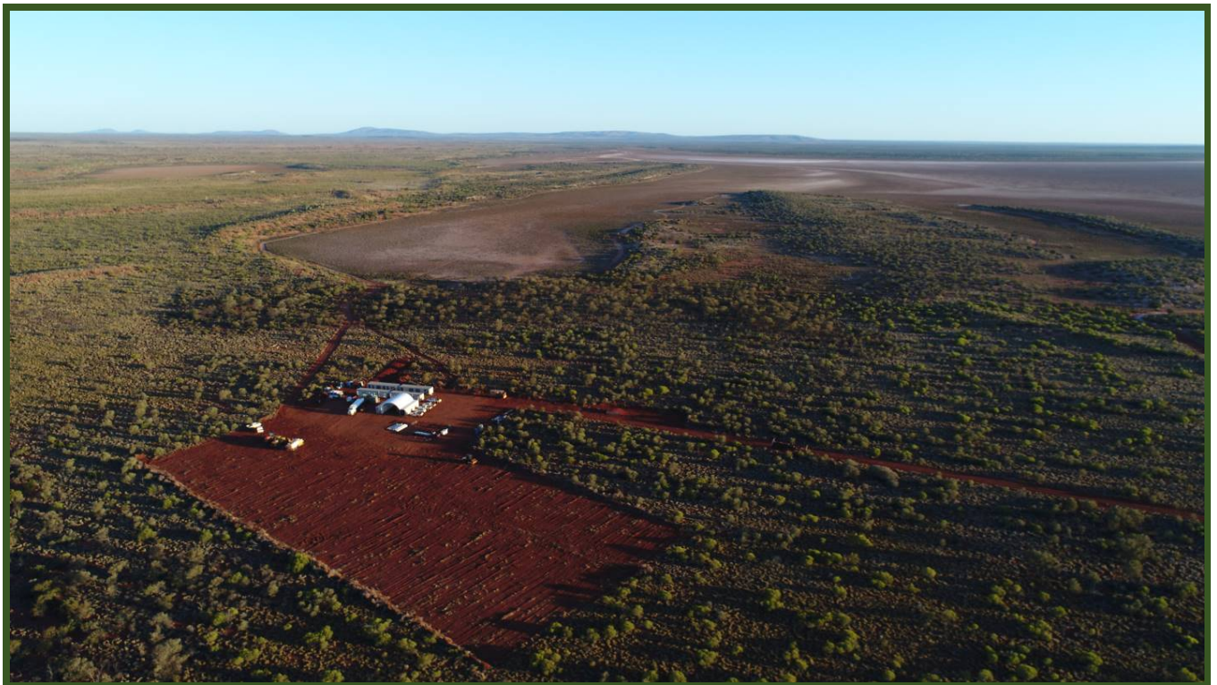
Beyondie Sulphate of Potash Project – Main Supporting Infrastructure Area
