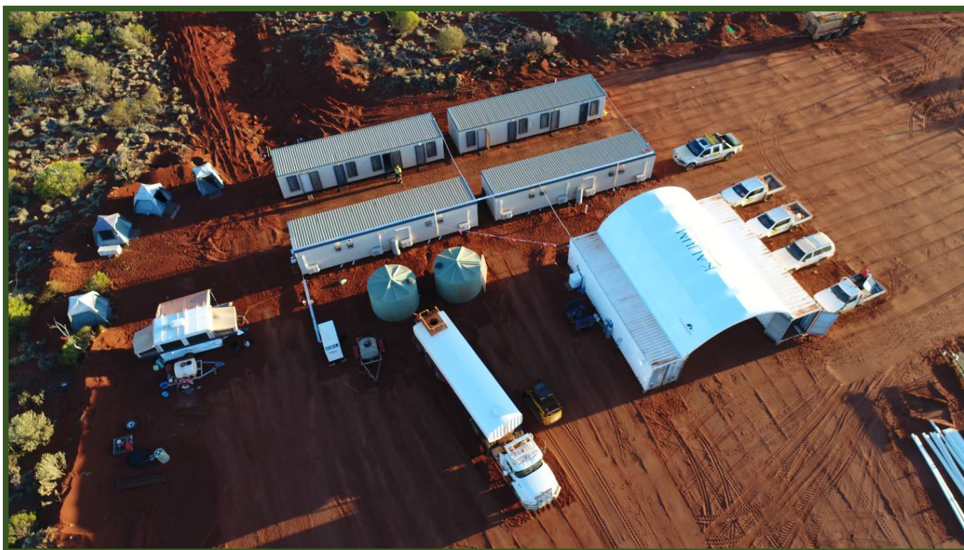
Beyondie Sulphate of Potash Project – Accommodation and Site Office Facilities
