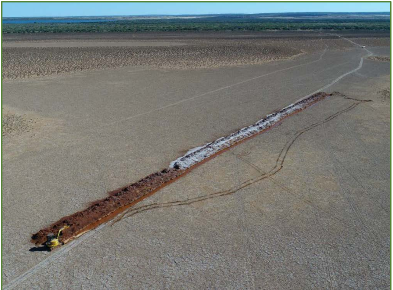
Aerial view of 10 Mile trench installation
