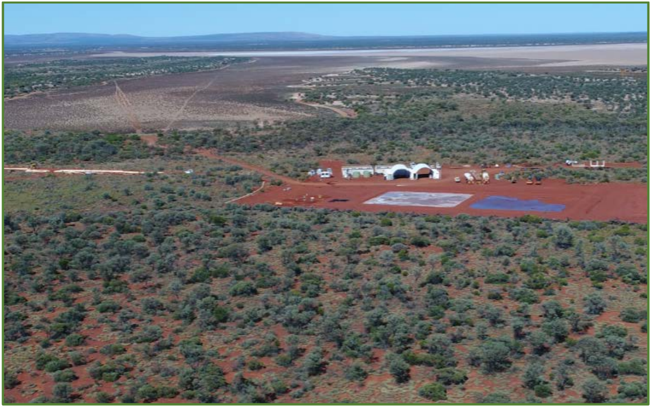
Aerial view of Infrastructure and Verification Ponds at 10 Mile
