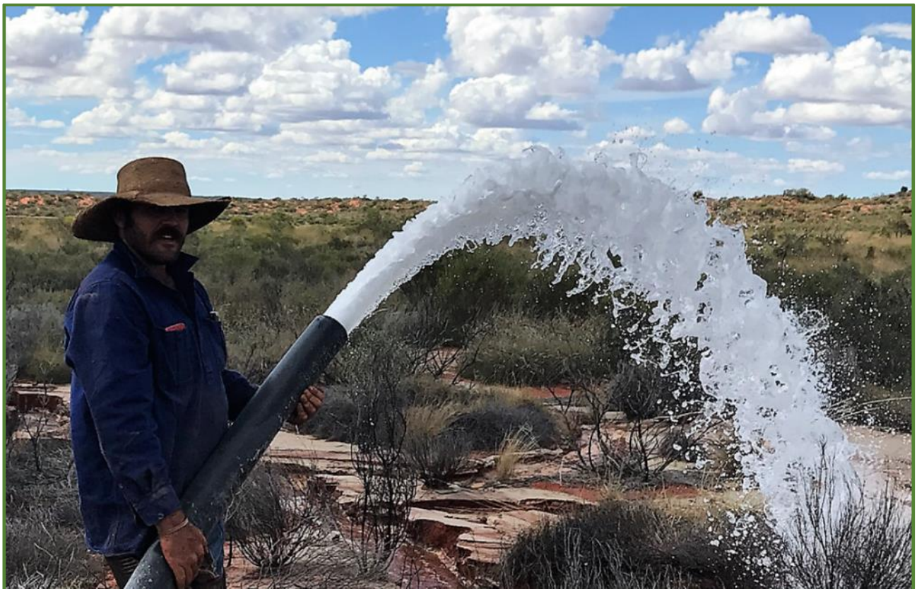
Brine Bore Test Pumping at approximately 27 litres per second
