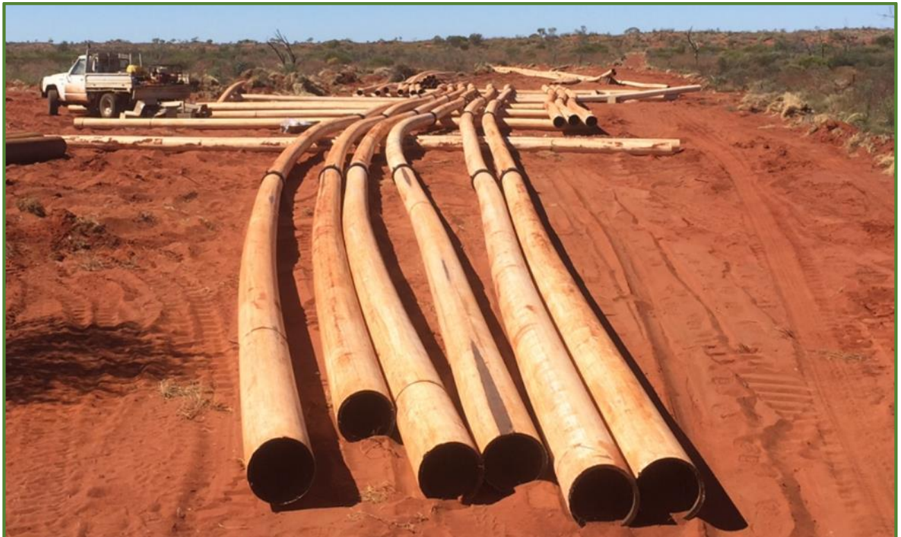
Pipeline assembly area at 10 Mile
