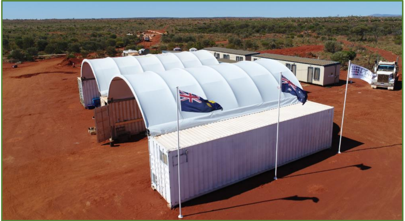
Workshop and Accommodation Facility at 10 Mile
