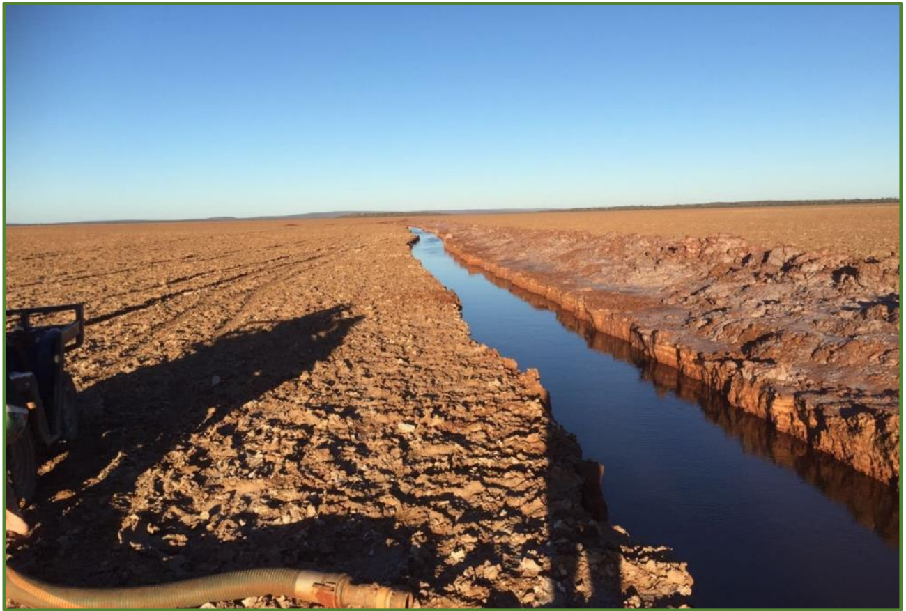
Trench installed at 10 Mile
