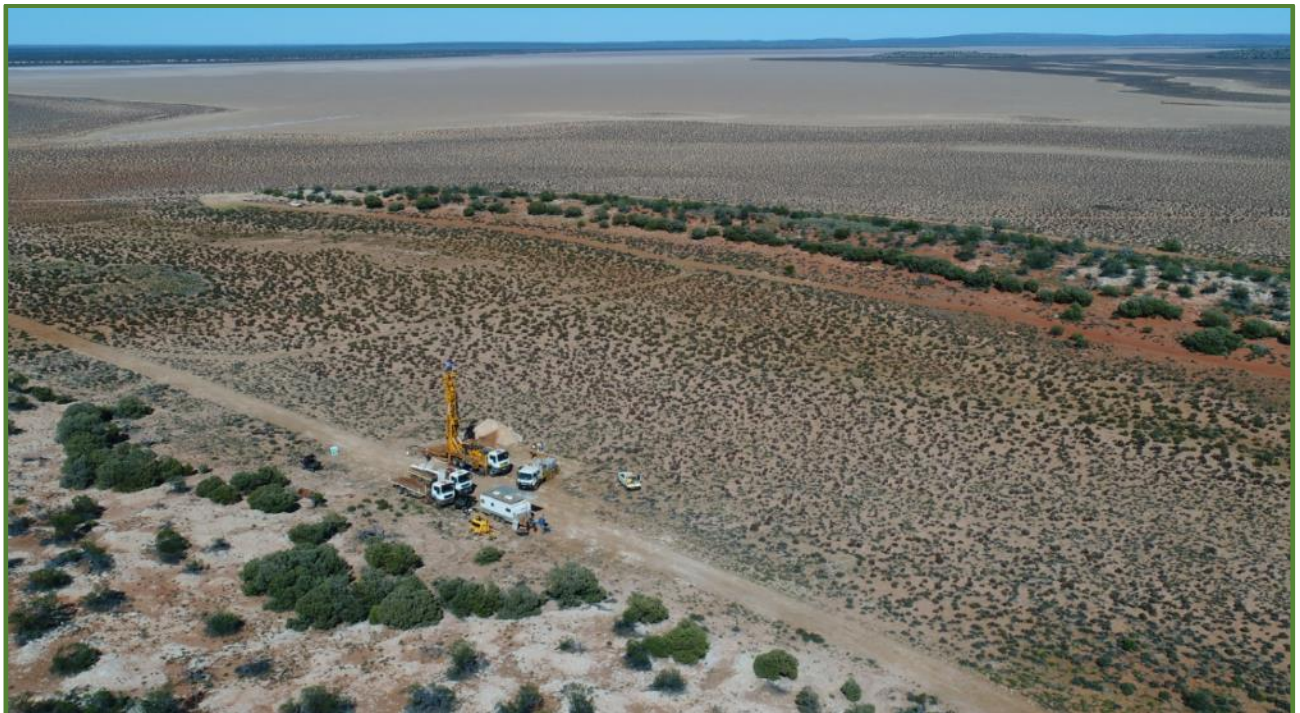
Drilling near 10 Mile
