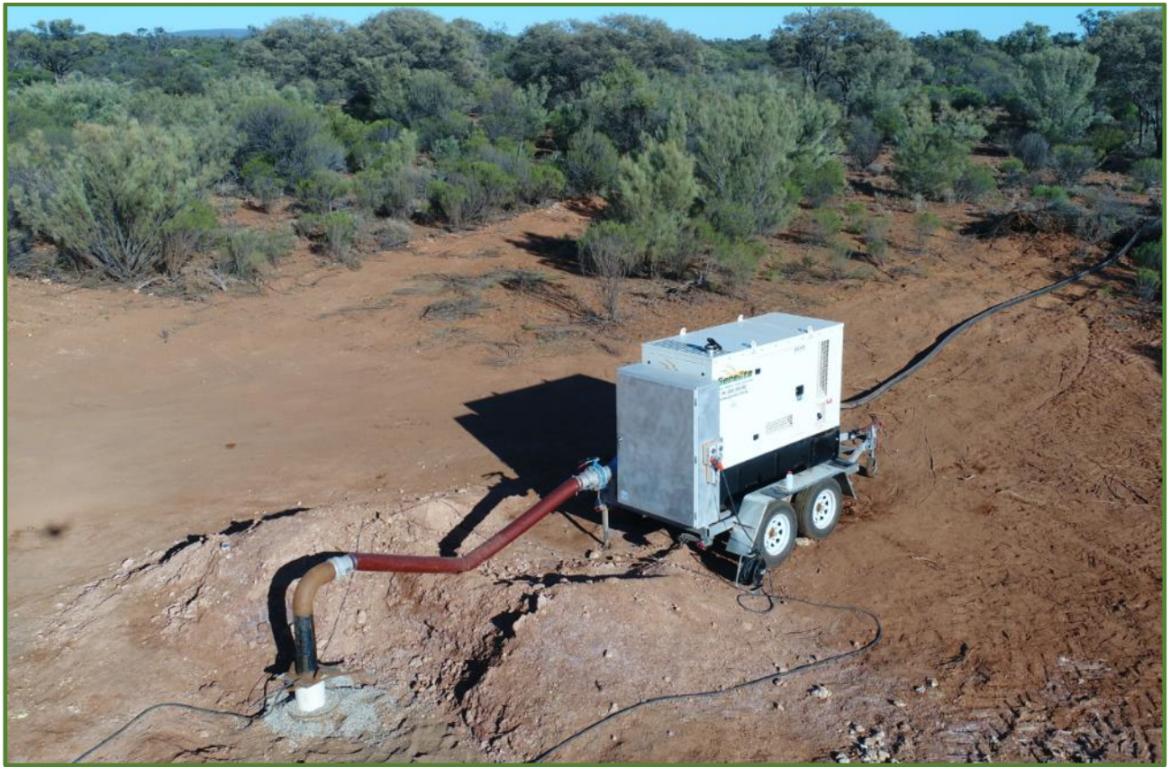
Test Pumping Rig and Production Bore Headworks
