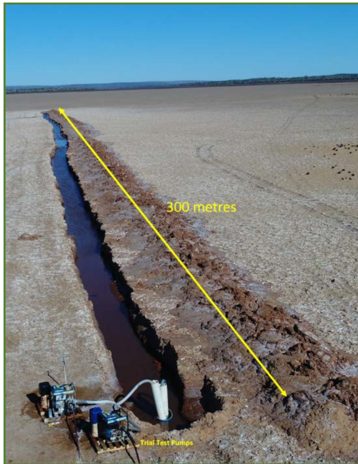
10 Mile Trench 2 Undergoing Test Pumping
