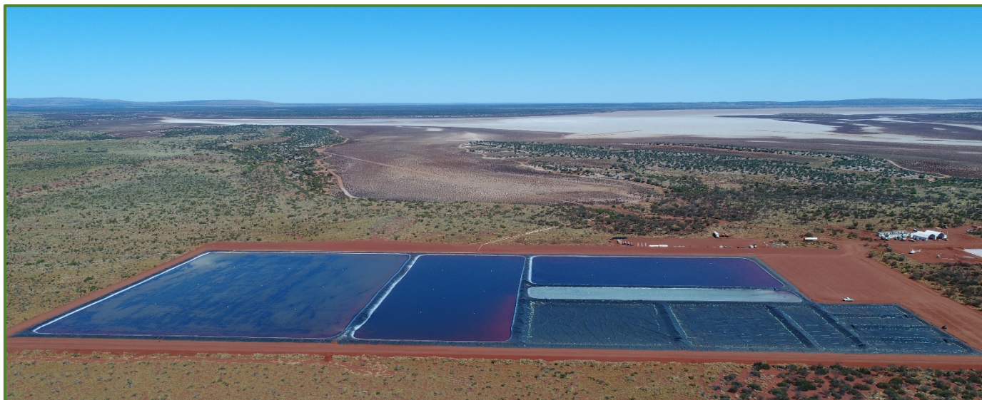
Continuous Gravity Flow - Large Scale Pilot Ponds
