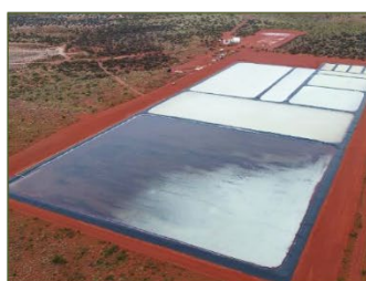
Brine Solar Evaporation Located in high evaporation region
