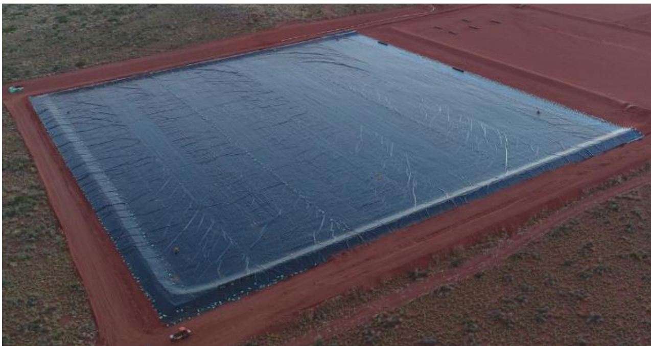
HDPE liner used for Large Scale Pilot Evaporation Ponds in 2017
