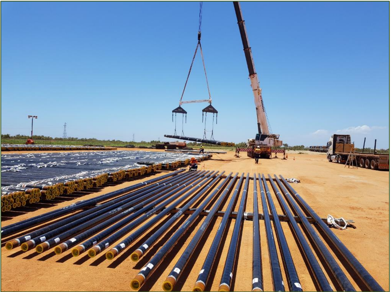
Gas pipe being prepared for transport from Port Hedland
