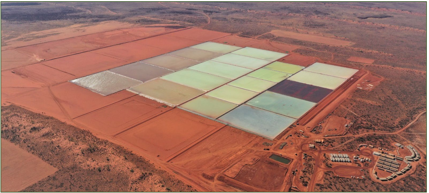
All Primary Potassium Crystallisation Ponds Complete and Operational – July 2020
