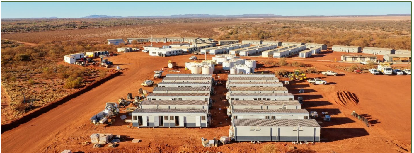
60 Additional Rooms for Construction Accommodation
