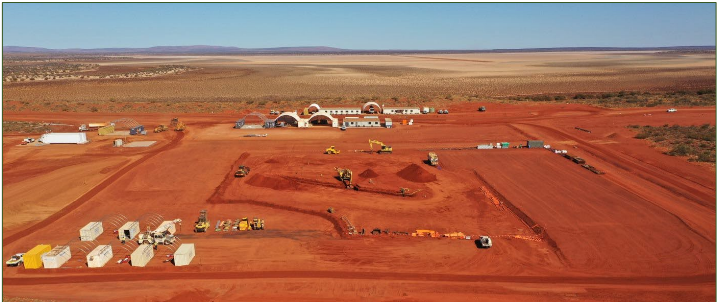
Construction of the SOP Processing Plant has commenced
