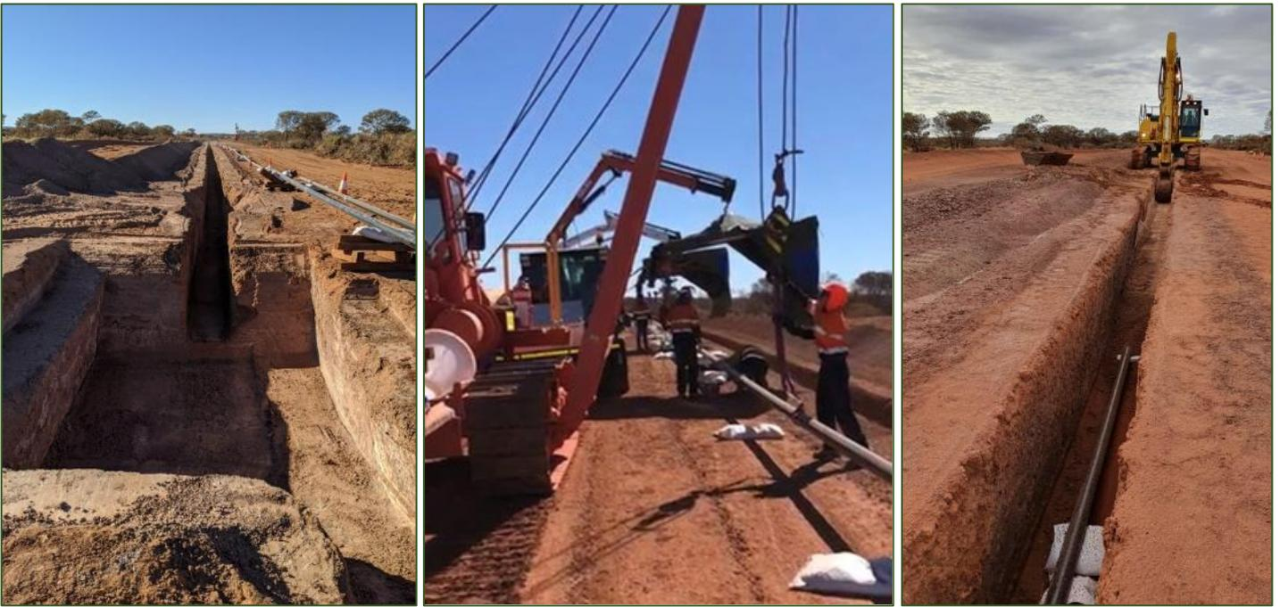
**Pipeline trench ready for pipeline installation (left), welding of the gas pipeline (centre) and pipeline installation (right)**
